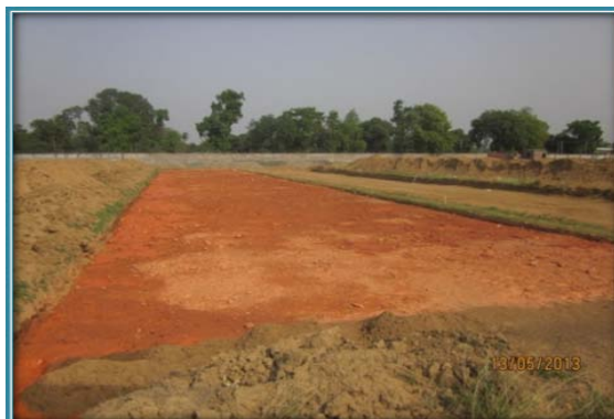
Road work in progress
