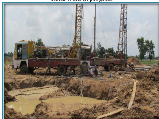
Rigs machine at work for Boys' Hostel
