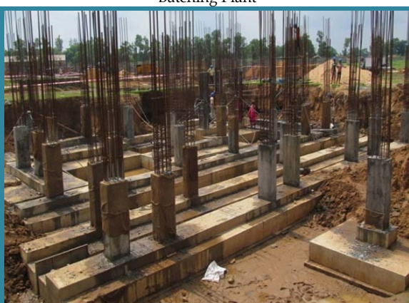
Foundation work in Academic Block
