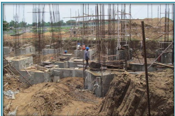
Foundation work of Theoretical Complex
